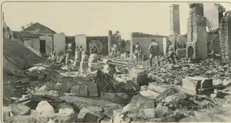
THE RUINS OF GOVERNMENT HOUSE, AT NICOSIA, CYPRUS, AFTER ITS COMPLETE DESTRUCTION AT THE HANDS OF A RIOTOUS MOB OF FIVE THOUSAND PEOPLE; A SEARCH AMONG THE WRECKAGE OF THE INTERIOR.
