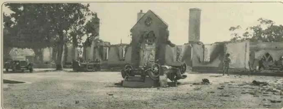
THE EXTERIOR OF GOVERNMENT HOUSE AT NICOSIA AFTER THE FIRE THAT DESTROYED IT WITH ALL ITS CONTENTS: THE RUINED WALLS OF THE FRONT, WITH SOME OF THE MOTOR-CARS, INCLUDING THAT OF THE GOVERNOR OF CYPRUS, WHICH WERE OVERTURNED AND BURNED BY THE MOB.
